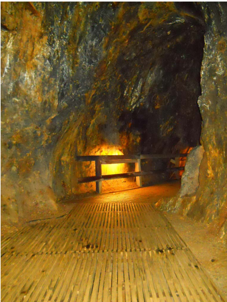
The underground workings of the Falun Mine. The walls are stained yellow due to sulfide mineralization of the area.
